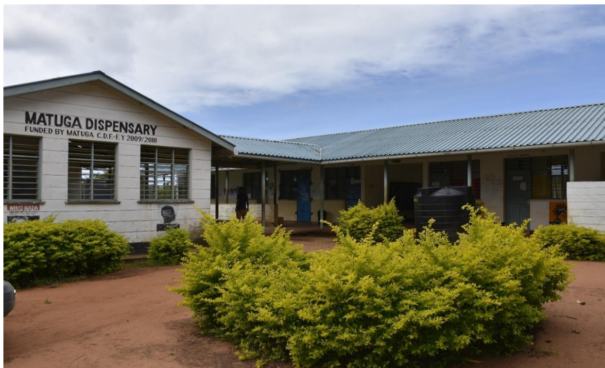
Figure 4: Photo of Matuga level 2 Dispensary.
